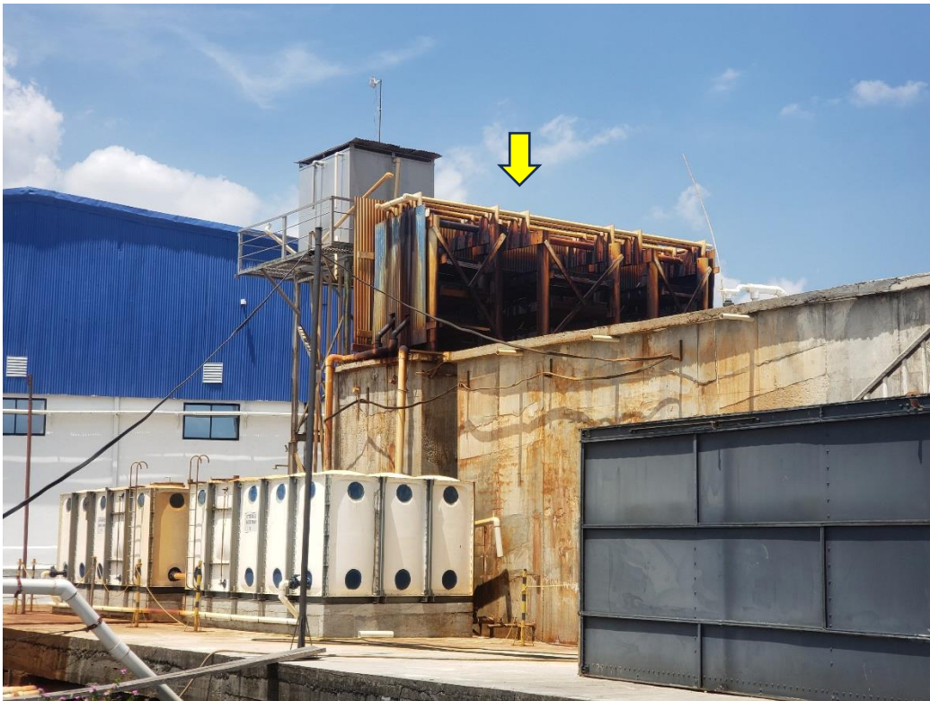
Figure 122: Aeration Tower – Water Treatment System
