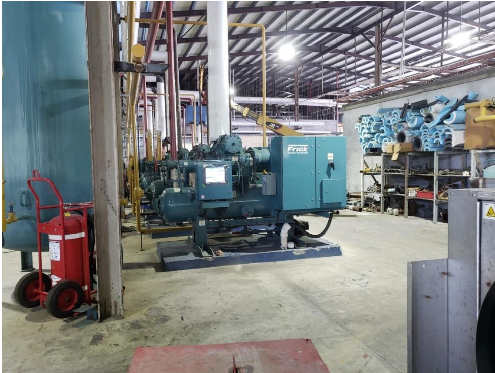
Figure 95: Low Stage Rotary Screw Compressors
