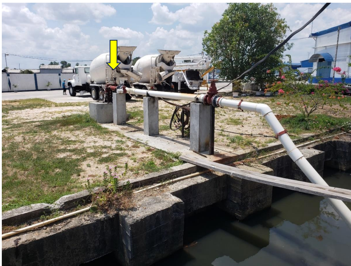
Figure 120: Artesian Well Head with outgoing supply lines
