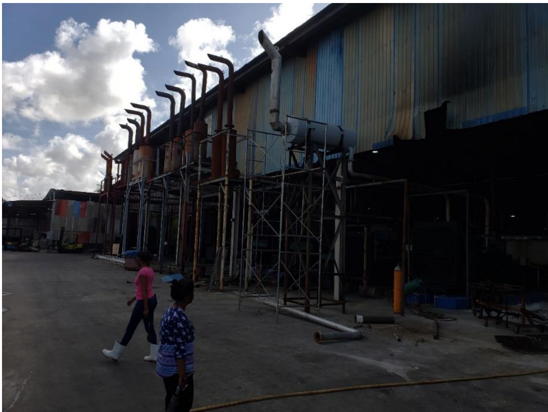
Figure 127: Muffler Systems with Stacks on Power Generation Units
